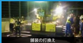
舗装の打換え
