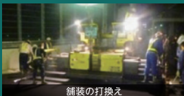
舗装の打換え
