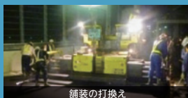
舗装の打換え
