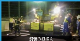
舗装の打換え
