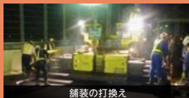
舗装の打換え
