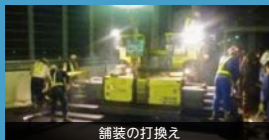
舗装の打換え
