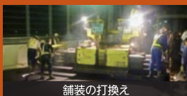
舗装の打換え
