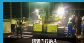
舗装の打換え
