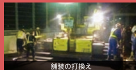
舗装の打換え
