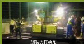
舗装の打換え
