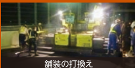
舗装の打換え
