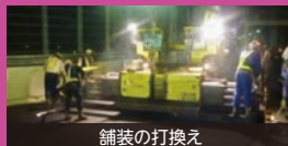
舗装の打換え
