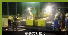
舗装の打換え
