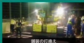
舗装の打換え
