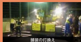
舗装の打換え
