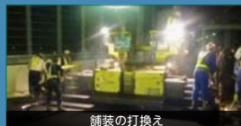
舗装の打換え
