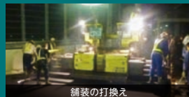
舗装の打換え
