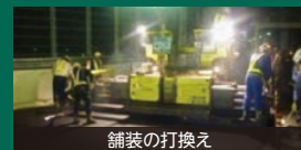
舗装の打換え
