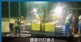
舗装の打換え
