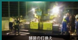
舗装の打換え
