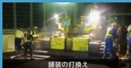
舗装の打換え
