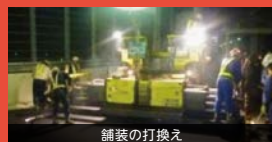
舗装の打換え
