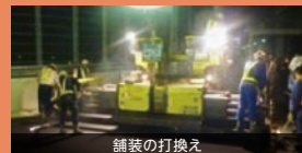
舗装の打換え
